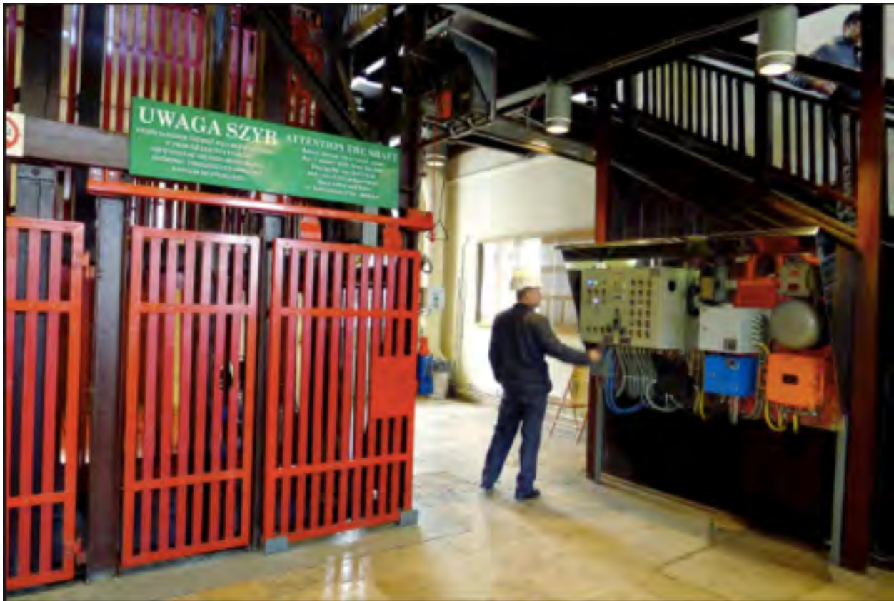
Elevator Cells in the Salt Mine
